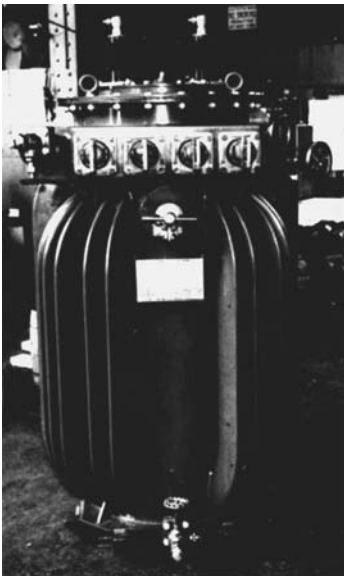
FIGURE 5.9 Medium-size transformer with corrugated tank.
