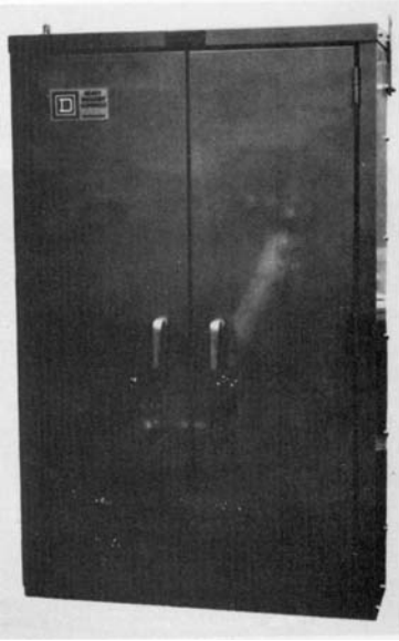
III. Time-current type in NEMA Type 4 (watertight) cabinet.
