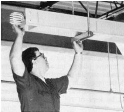
FIGURE 9.163B Installing busway on hangers.
