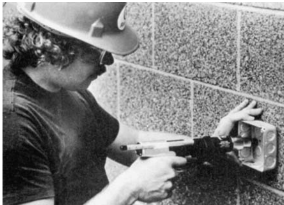
FIGURE 4.230 Ram-Master semiautomatic power-load feed assembly. [Ramset, Olin Corp.]
