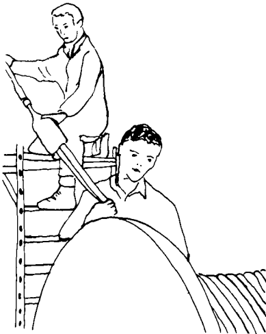
FIGURE 2.52 When bare steel basket grips and similar pull-line-to-cable devices must be used, cover them with plastic tape or rubberlike shields.
