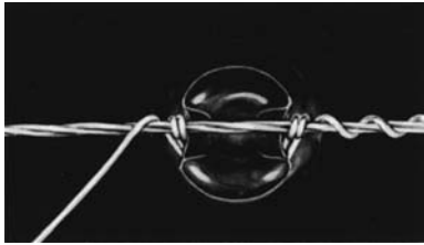
V. Complete six spiral 45° wraps on each side of the insulator, bending back the ends and cutting them off short.
