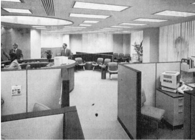
FIGURE 10.97 Illumination with large-area fluorescent ceiling units.
