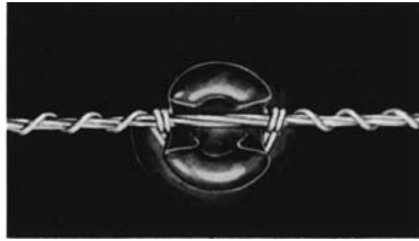
VI. The finished top tie when made properly and tightly will greatly reduce any possibility of the conductor's chafing at the insulator.
